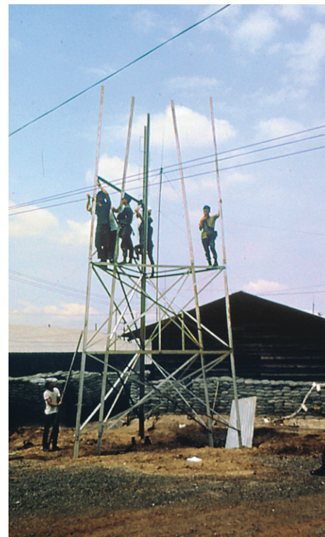
The Army of the Republic of Vietnam's 1st Engineer Group is trained to erect a Bilby tower by the 66th Topographic Company.
