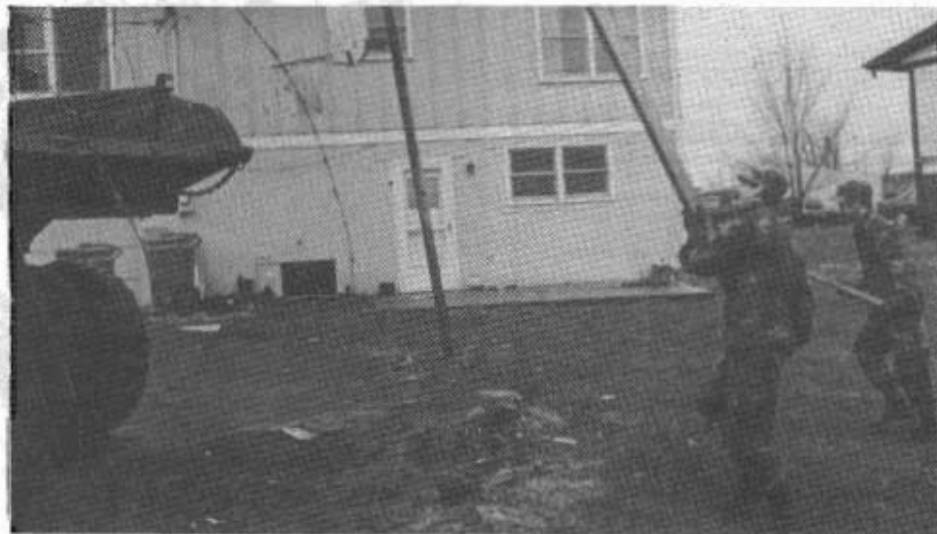
Clean-up operations in Lexington brought out members of Company D, 201st Engineer Battalion from Carlisle. Sgt. Jon R. Tedder (left) and SP4 Edwin Purvis remove debris from the backyard of a home damaged by the severe weather. (photo by Capt. Frank Mattingly)
