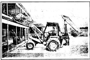
The front bucket of Spec. Charles H. Hannah's backhoe is used to catch waste from the remodeling work on the second floor of the Annex.
