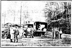
MOBILE WATER PLANT -- The 217th QM DET's purification system set up at the Wheelwright community pool produced 90,000 gallons of potable water.
