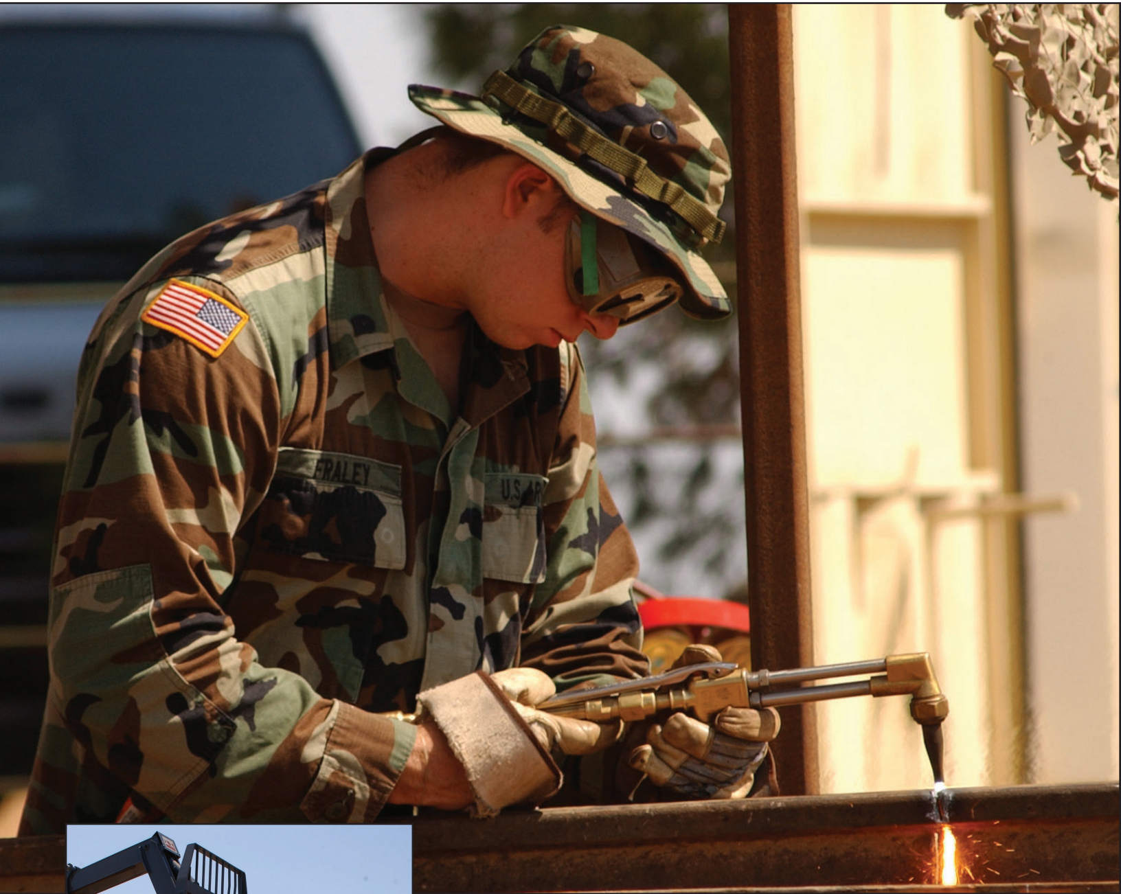
Spec. Tony Fraley, Bravo Company 206th Engineers cuts a steel beam that will be welded into a temporary vehicle barrier in Sasabee Ariz. along the Mexican border.
