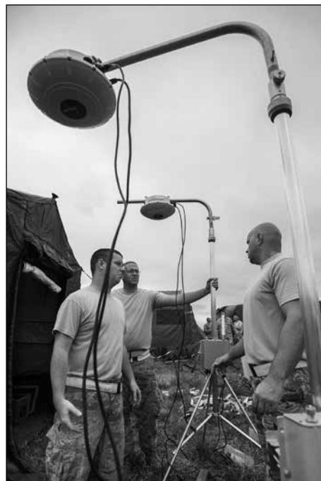
Airmen from the 123rd CRG assemble Radio Frequency Identification gear, used to wirelessly track cargo and equipment, at MidAmerica St. Louis Airport Aug. 5.
